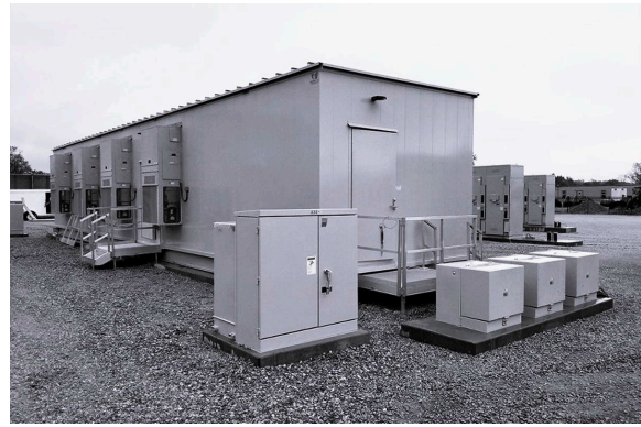
Power transformer. Source: CAT, 2017.
