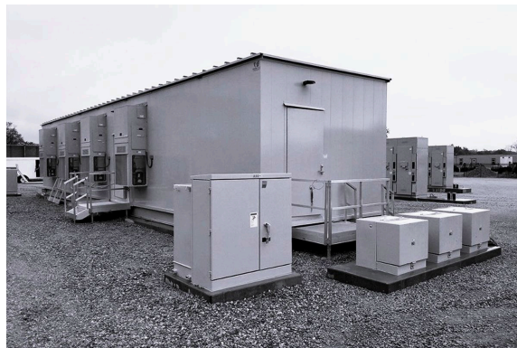
Power transformer. Source: CAT, 2017.
