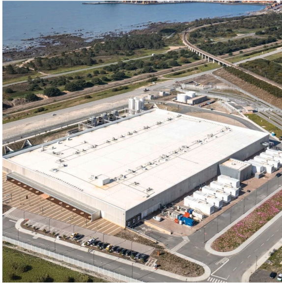
SINES Data Campus. Source: startcampus.pt, 2025.
